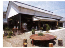
Exterior of a building once used as a sake brewery
